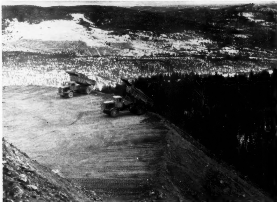
WASTE DUMPS are built up adjacent to the open pit. Here are two Euclids dumping into a steep ravine. Average waste haul was 1,100 feet. The steep hillside which rises from the 3,200 foot bench to the 4,260 bench made it possible to establish several dumps to dispose of the plus-2,000,000 cubic yards of soil gravel and the 1,500,000 cubic yards of rock waste.
